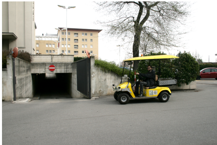
Fig. 16. Garage ramp of the U5 building (picture taken from the external parking lot).
