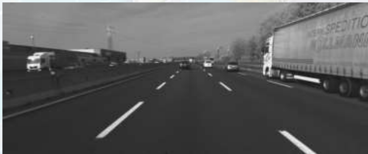
A4 Highway, Milan-Bergamo, Italy 4-Lanes Configuration
